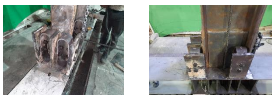
Fig. 9. Instalation and placement of CFD dampers
