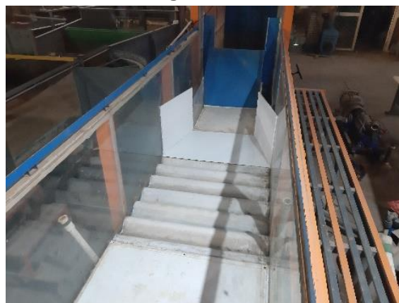
Fig. 5. A view of corrugated bed and expansion
