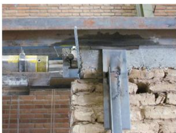
Fig. 13. Initiation of diagonal cracking
