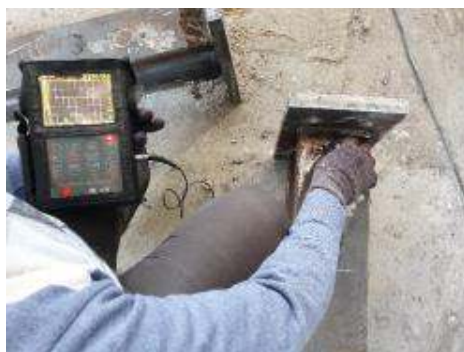
Fig. 2. CJP Ultrasonic Weld Test
