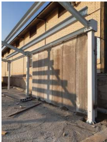
Fig. 12. Installation of the perimeter walls
