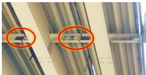
Fig. 3. Removed lateral connections between girders
