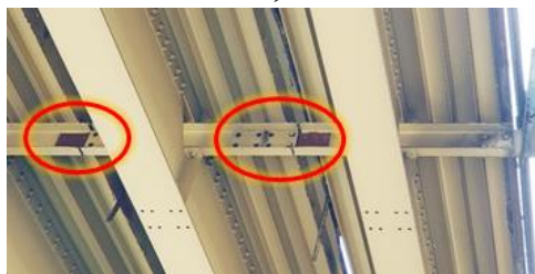
Fig. 3. Removed lateral connections between girders
