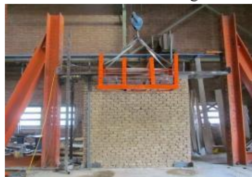
c) Overall view of the wall
