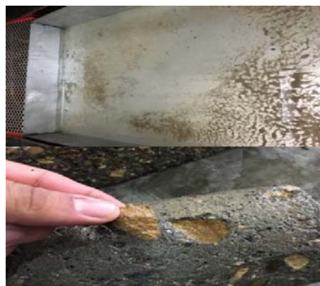
Fig. 3. Detachment of aggregate after 300 cycles
