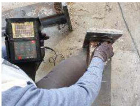
Fig. 2. CJP Ultrasonic Weld Test
