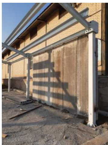
Fig. 12. Installation of the perimeter walls
