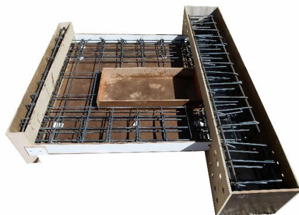
Fig. 4. Formwork of specimen
