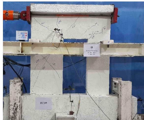
Fig. 8. Cracking pattern on drift 1.34%
