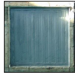
Fig. 10. Exposed surface of PIR SWP-M3 after test
