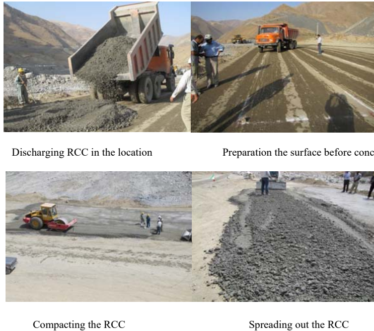
Fig. 8. Images of the Test Pad Construction
