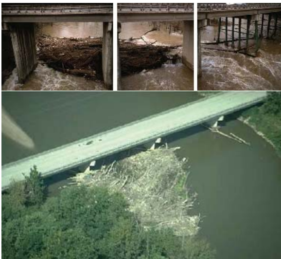
Fig. 1. The accumulation of driftwoods in bridge span and the phenomenon of flow obstruction
