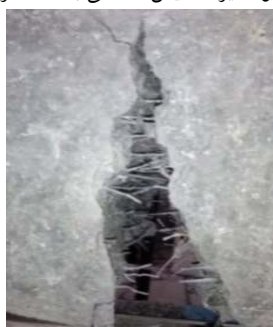
Fig.20. bending beam Sample after failure
