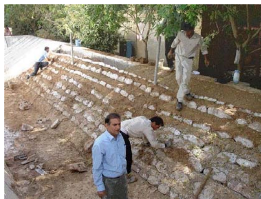
Fig. 1. General view of experimental set-up
