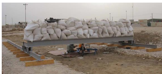
Fig. 2. Photo of the cart and modular rails system on the prepared embankments.
