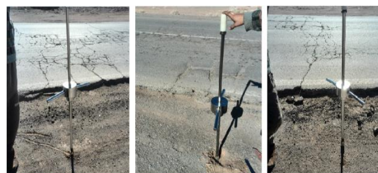
Fig. 1. DCP test at different points of road in field.
