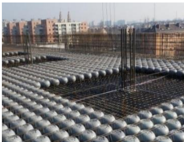
Fig. 1. A view of the implementation of the ceiling of the bubble slab
