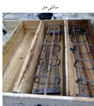
Fig. 2. Molding and reinforcement placing for the specimen
