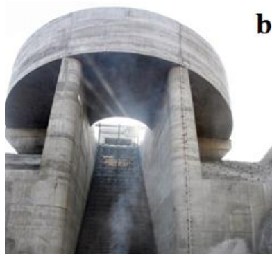
Fig. 2. Khoda-Afarin dam a: Plan view b: Modern horseshoe spillway and hydroelectric power plant intake (Ref.: www.Taminrah.com )
