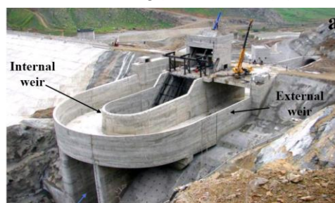
Duct for hydropower plant's intake and Internal weir
