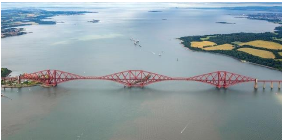
Fig. 12. The forth bridge
