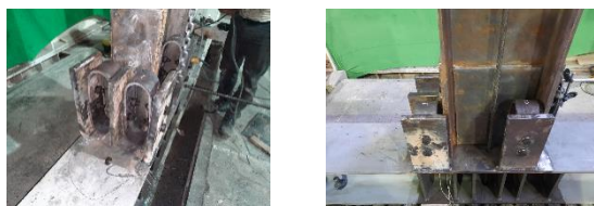
Fig. 9. Instalation and placement of CFD dampers
