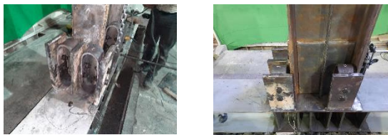
Fig. 9. Instalation and placement of CFD dampers
