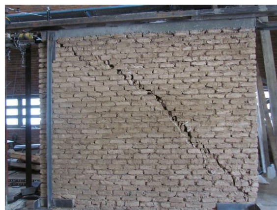
a) Front view of the cracking in the wall
