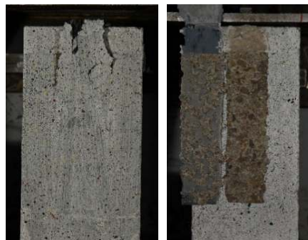
Fig. 6. Different failure modes
