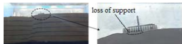
Fig. 9. Foundation reinforced with one layer of geogrid
