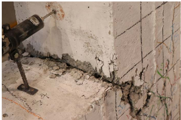
Fig. 10. The crack of the joint at 6% drift of TDN sample
