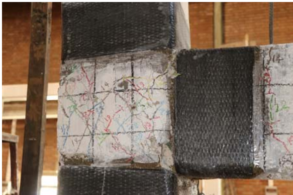
Fig. 22 Beam column joint after the test in TDS sample
