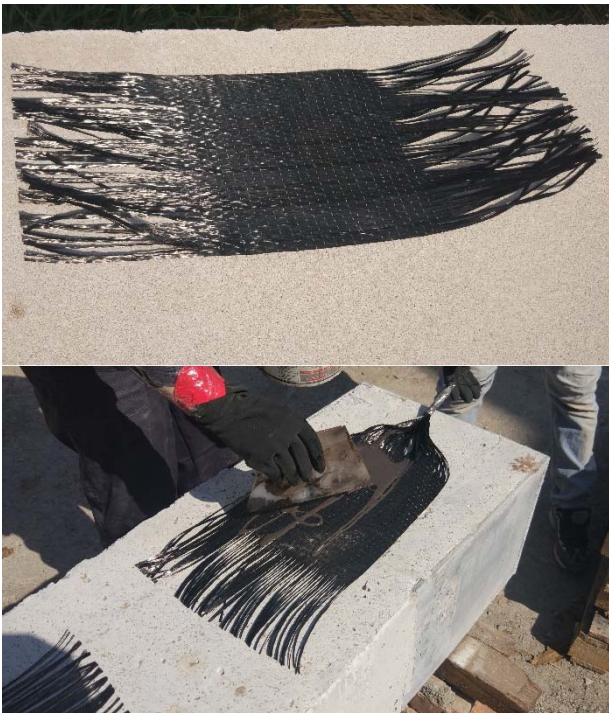
Fig. 3. Preparation of FRP anchor (top picture) and impregnate it with resin (bottom picture)
