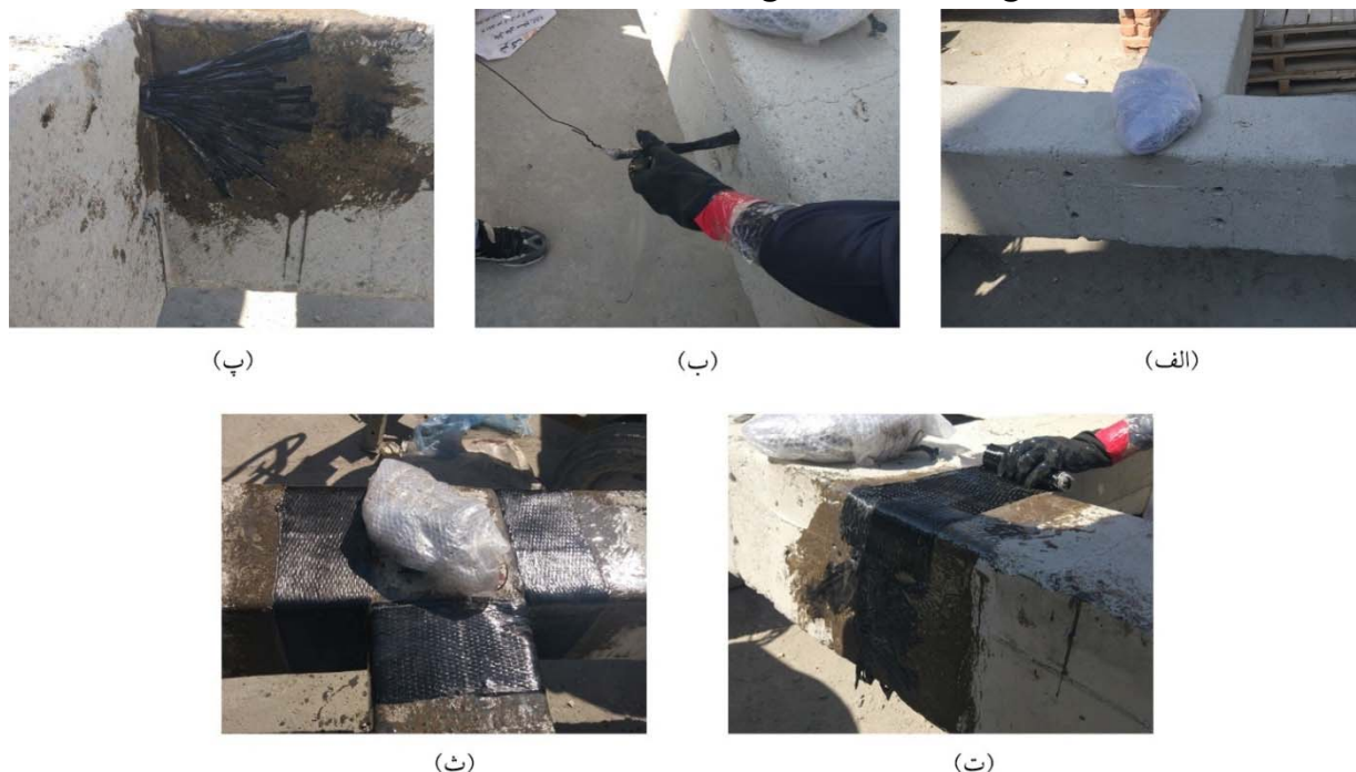
Fig. 5. Preparation and retrofitting of TDS sample with FRP : a) preparation of the surface and piercing, b) pass the FRP dowel through the holes, c) pasting FRP to the surface, d) pasting strips on the dowels, e) the specimen after retrofitting with FRP
