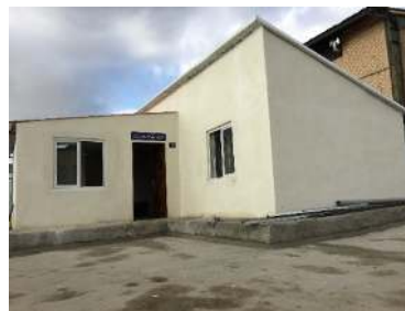
Fig. 13. The completed proposed pre-fabricated building with the assemble and disassemble abilities
