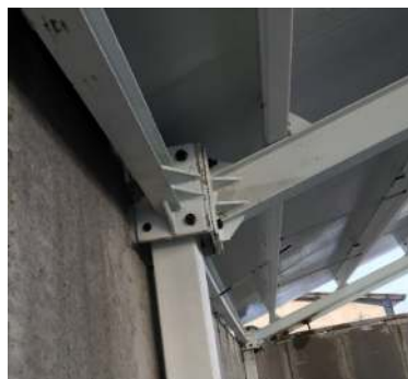
Fig. 11. A close-up view of the fabricated proposed beam-to-column connection
