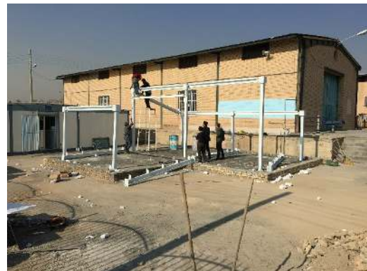
Fig. 9. A view of the frame installation process: Installation stage of the beams and columns
