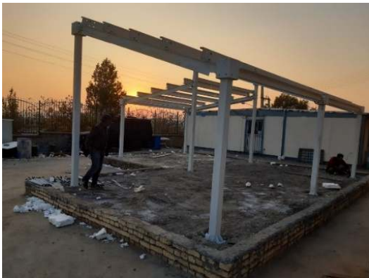
Fig. 10. A close-up view of the frame installation process: Complete installation stage of the skeleton
