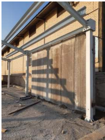
Fig. 12. Installation of the perimeter walls
