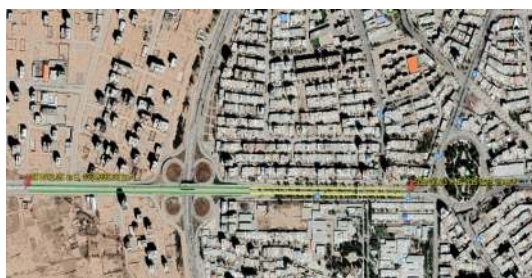
Fig 10. Location and quality condition of pavement sections (Kowsar Blvd)
