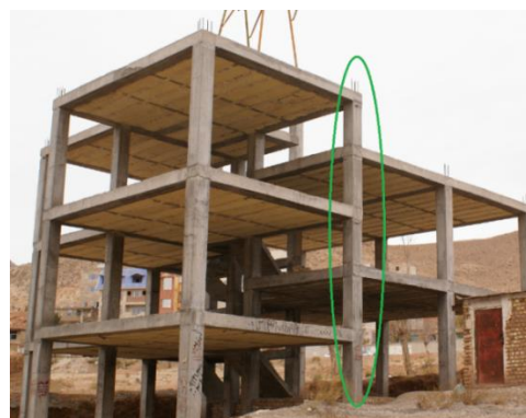
Fig. 2. The short columns in a duplex building
