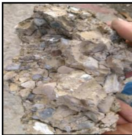
Fig. 4. A concrete sample taken from Plasco debris before fire resistance test.
