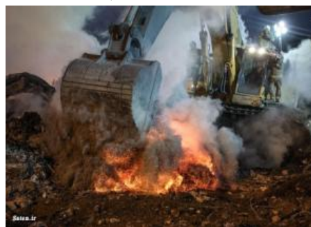
Fig. 3. Melted pieces during debris removal
