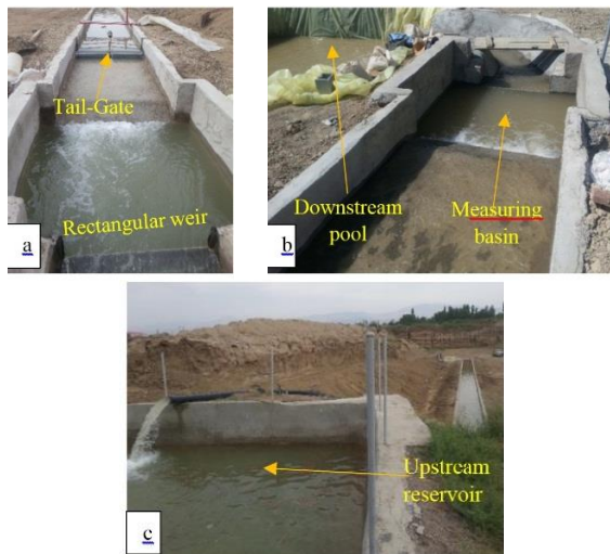
Fig. 3. (a) Rectangular weir and tailgate (b) measuring pond and downstream pool (c) upstream pond
