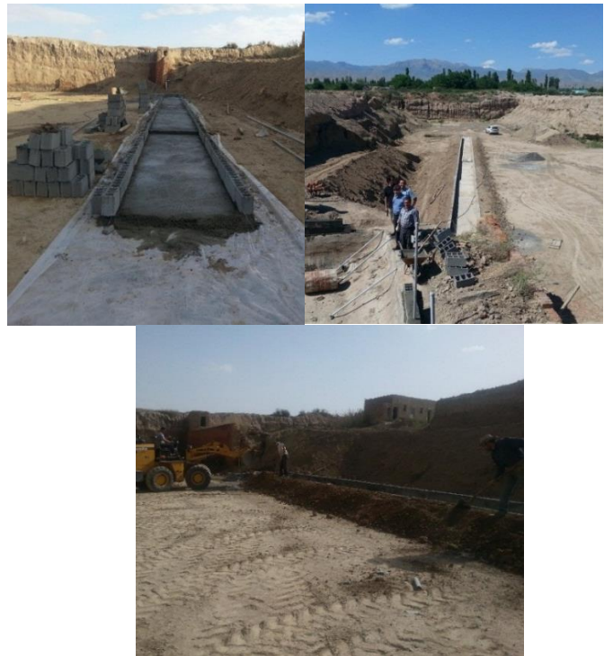
Fig. 1. Construction of physical model of a wide channel.
