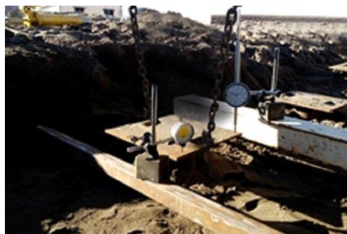
Fig. 1. The distance of installed piles in soil and application of displacement dial gauges
