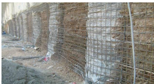
Fig. 3. Cast in place concrete piles along the northern pit wall
