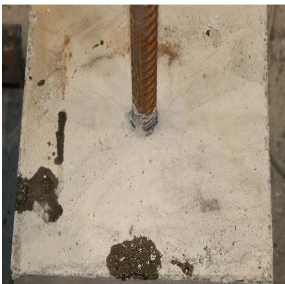
Fig. 7. Picture of pulled out rebar (P25S1)
