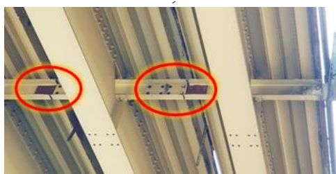
Fig. 3. Removed lateral connections between girders
