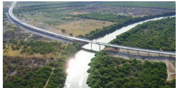
Fig. 1. Rio Grande Bridge, Mexico
