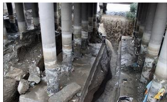
Fig. 2. Bridge Failures due to Scour (Kan Bridge)
