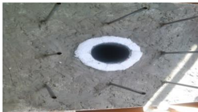
Fig. 5. Protected tube with 40mm thickness geofoam
