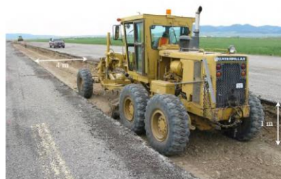
Fig. 1. The filed test trench [23]
